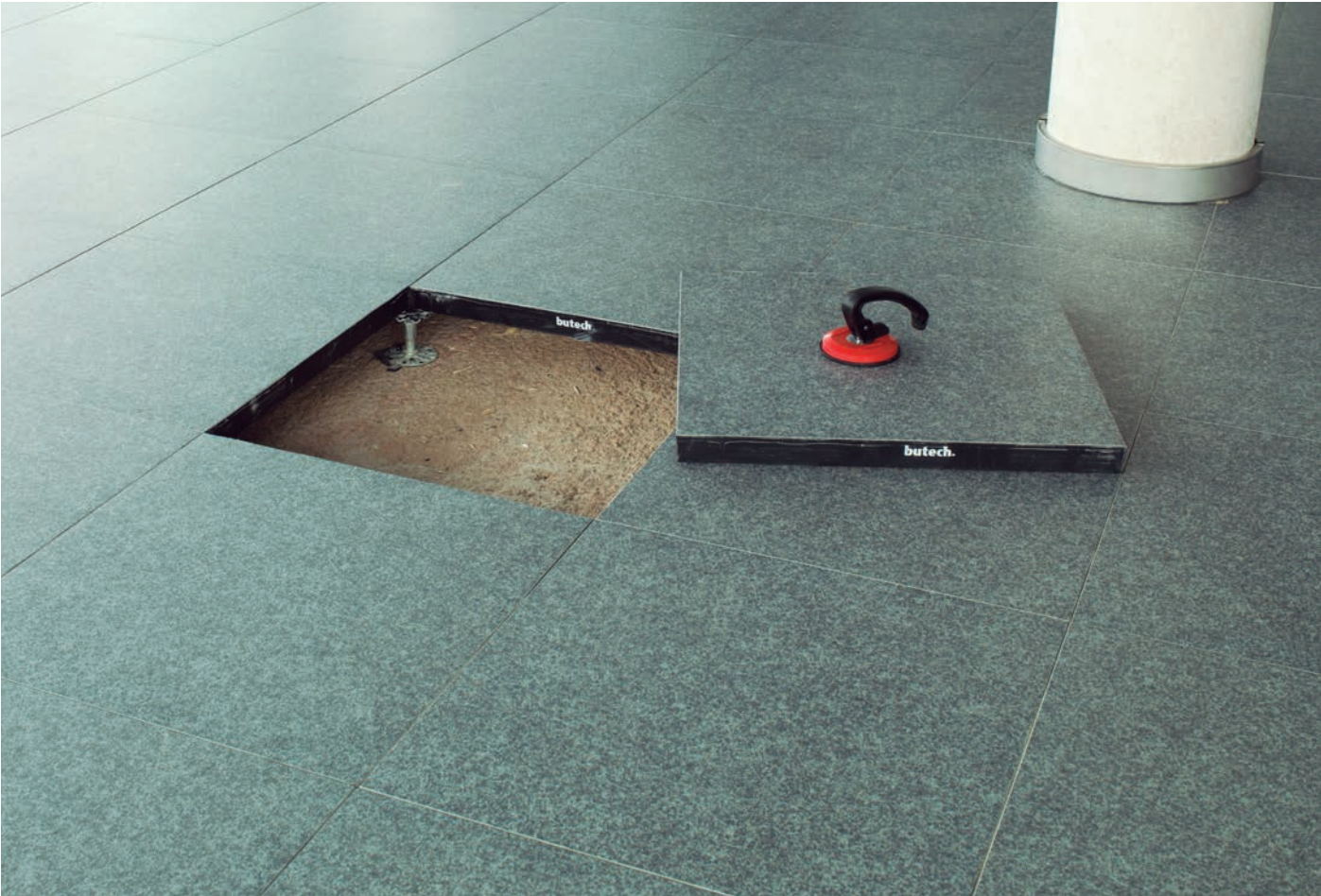
Technological building of UJI University (Castellón, Spain)
