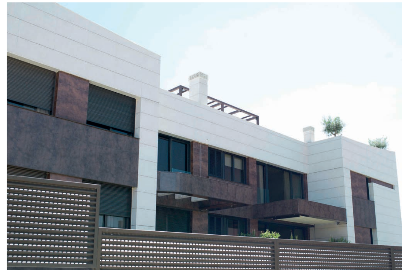
Residential building (MAdrid - Spain)
